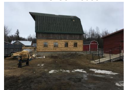
Barn being refurbished
