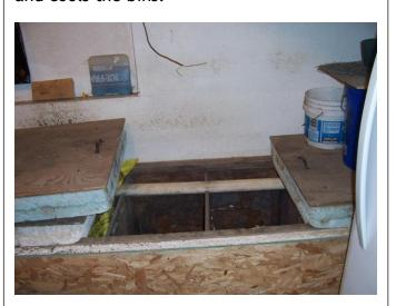
This photo gives you an idea of the construction details. Four inches of foam is a good insulator. The lids are light in weight and can give access to the bin desired without removing the whole top.
