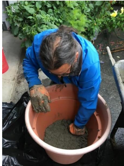
Adding the cement mixture into the form - the cement mixture is slowly built up inside, 1 - 2 inches thick.
